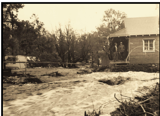
The next morning, west side of the Monterey Trail bridge
