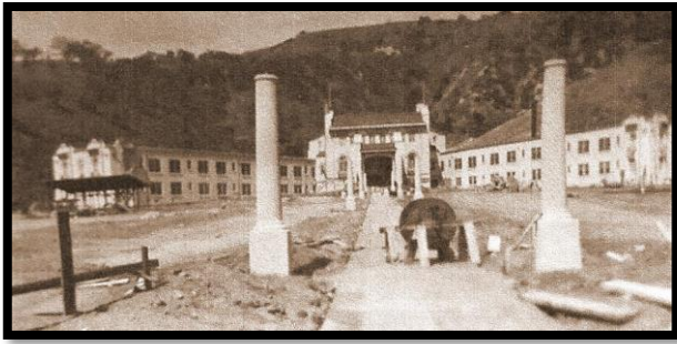
The Lebec Hotel under construction
